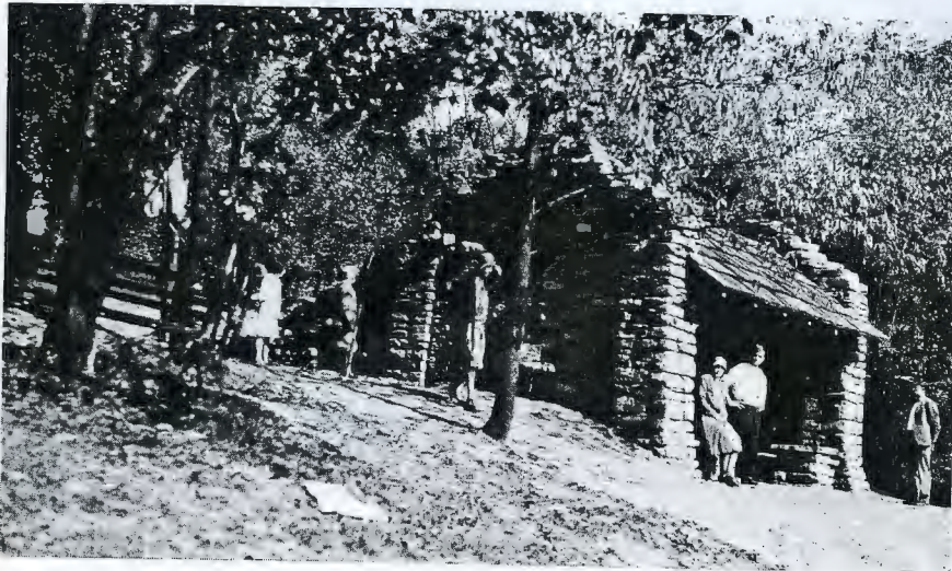
THE MOUNTAIN TYPE OVEN SHELTER WITH OVENS ON TWO LEVELS, ONE UNDER COVER, THE OTHER OUTDOORS
