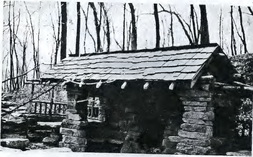
ON THE SIDE OF AN OLD QUARRY
