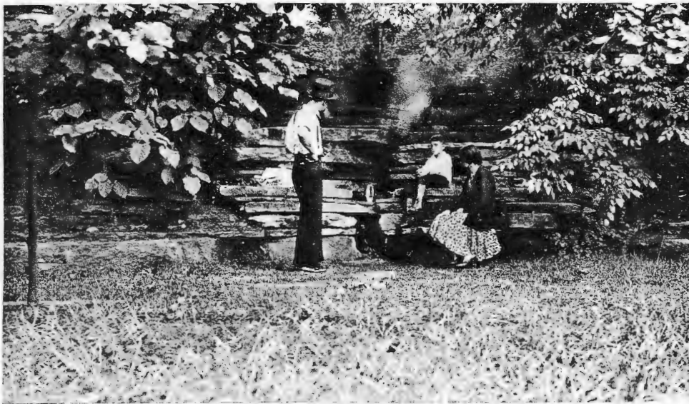
ROCK STRATIFICATIONS ARE ALWAYS OF INTEREST IN THE LANDSCAPE. HERE THEY HAVE BEEN COMBINED TO FORM A CAMP OVEN, COMPLETE WITH SHELVES AND SEATING ARRANGEMENTS, AND SIMULATED OUTCROPPINGS. YOU GUESSED IT, THE CREVASSE IS NOT THE CHIMNEY, WHICH IS INVISIBLE AND LOCATED TWO FEET TO THE LEFT
